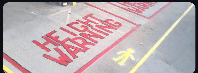
Height warning markings, loading bay
