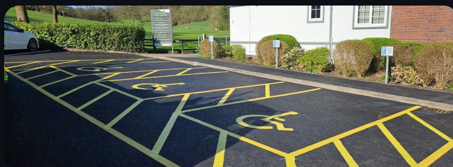
disabled parking bays
