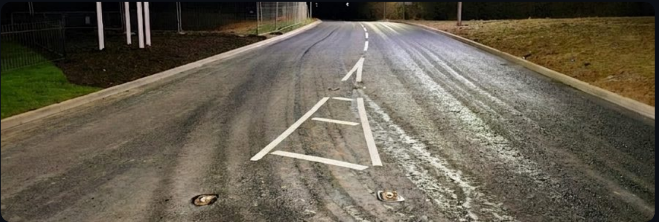
highway/civil works - Thermoplastic road markings
