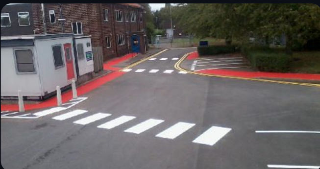
coloured walkways - zebra crossings
